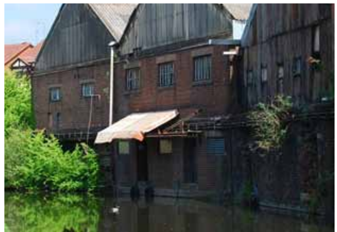
The New Dial Glass Cone and the remains of barge canopies Mike Jackson © RGS-IBG Discovering Britain
