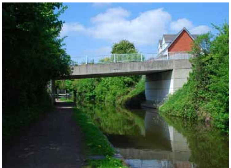
Longboat Lane Bridge Mike Jackson © RGS-IBG Discovering Britain
